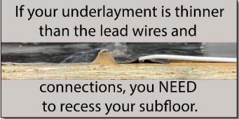
If you need to channel into a concrete subfloor, this must be done prior to installing your vapor barrier and underlayment. Refer to your planned layout to determine where power supply lead wires will route to the junction box. Remember the lead wires cannot run underneath any of the heating mats. Use a grinder tool such as an angle grinder or rotary die grinder (Dremel) in a concrete subfloor.
