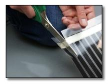
Make a cut across the silver metal conductor bar one black heating element from the end of the mat. Do not cut into black heating element bar as this will cause the GFCI to trip. Do <u>not</u> cut through the white skrim on the top and bottom of the mat.
