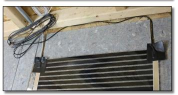
Push the cold leads and connectors down completely so the tops are level with the mat.
