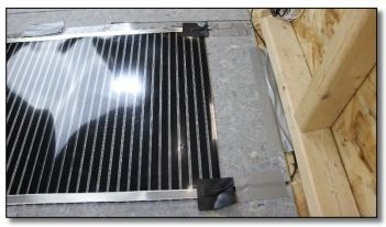
Use duct tape to secure in place.
