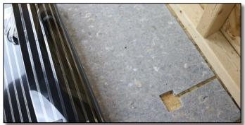
If you used an underlayment, cut a channel for the power supply lead wires and connections out of the underlayment. If there is a vapor barrier below your underlayment, be careful not to cut the vapor barrier.
