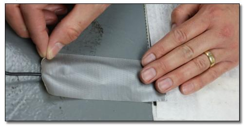
We do not recommend overlapping the mats, however if mats need to placed close together for layout, you must ensure no portion of the silver or black heating elements, or the electrical connections or wires should be overlapped.
