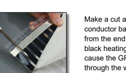
Make a cut across the silver metal conductor bar one black heating element from the end of the mat. Do not cut into black heating element bar as this will cause the GFCI to trip. Do <u>not</u> cut through the white skrim on the top and bottom of the mat.
