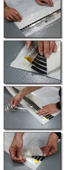
Fold back and crease the top white "flap" on the side of the heating panel to keep it out of the way while working with the bottom flap.
